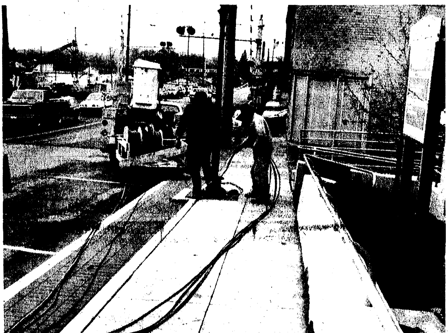
WIRE had to be fished through underground conduit in order to provide power to the new downtown old-style street lights, which have been installed on the east side of Main St. and part of the west side.
